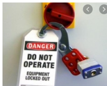
Fig.4. Electrical Lock-out system
