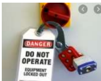
Fig.4. Electrical Lock-out system
