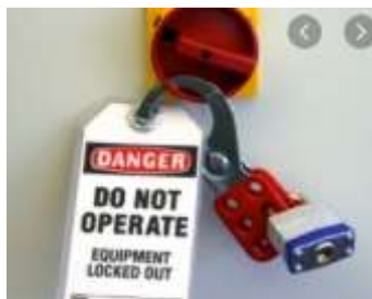
Fig.4. Electrical Lock-out system
