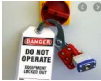
Fig.4. Electrical Lock-out system
